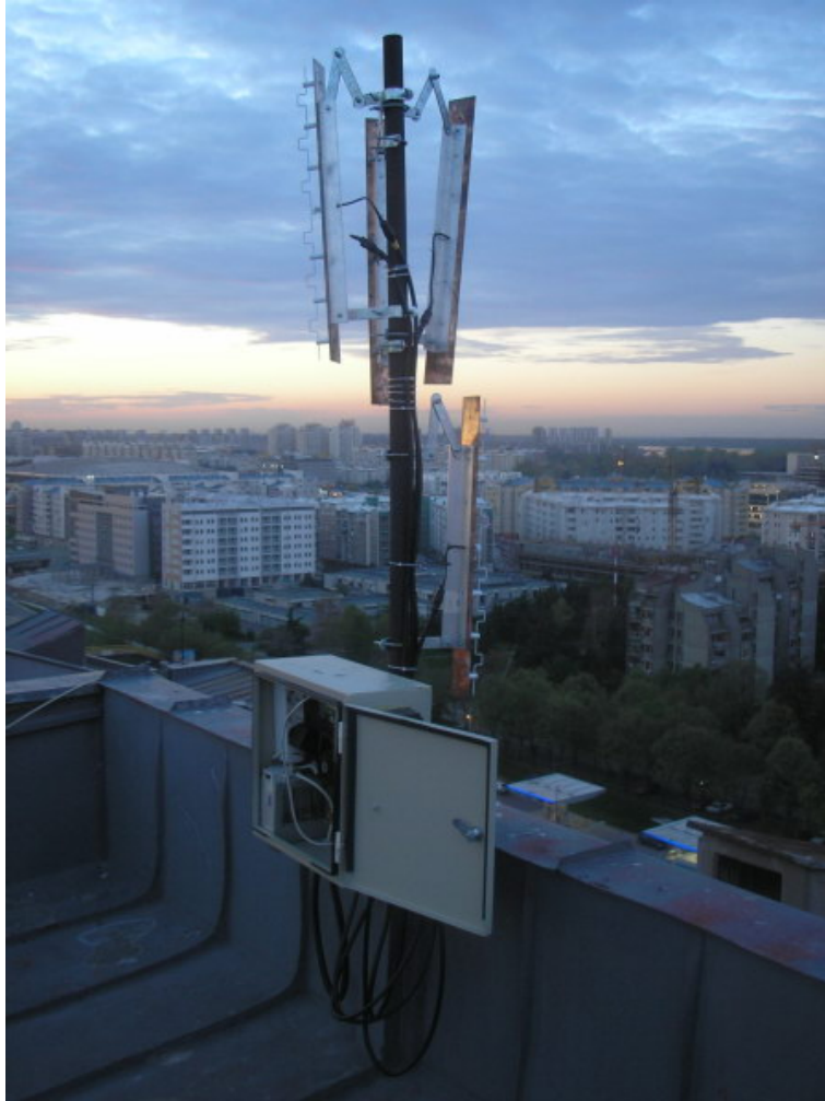
Fig. 18. Inverted Amos antennas with 7 dipoles at WLAN Access Point location.
